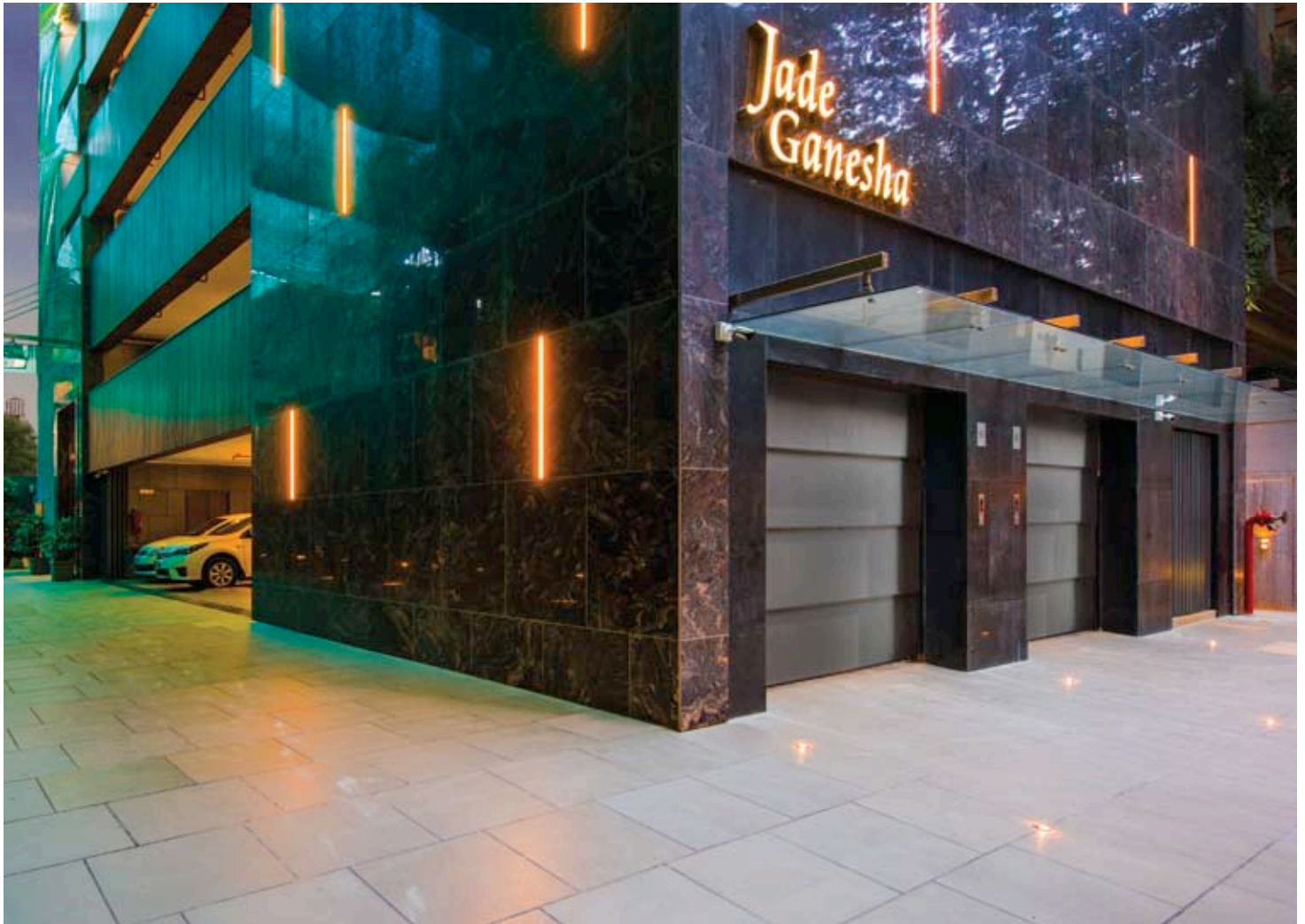
GA design achieved 60% savings in total power consumption by using highly energy-efficient LED lights in the common areas of the building.
